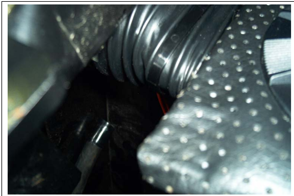
Install flex for upper vent to evaporator box.
